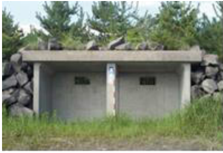
[退避壕設置事例(桜島)]
